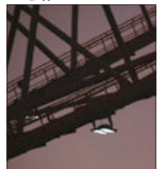
A Phoenix Products' floodlight in a mining application
